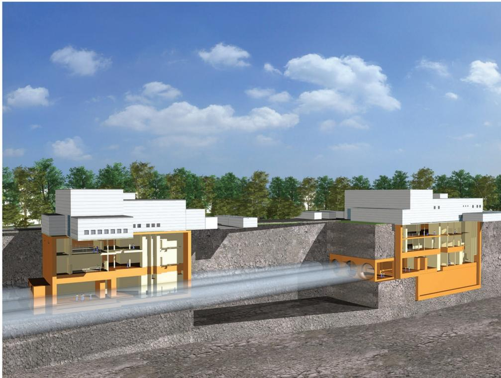
**Figure 7.1.24** Three-dimensional view of the shaft complex XS1 and XS5 at the XFEL site Osdorfer Born.
