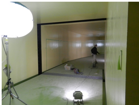
Inside DR tunnel
