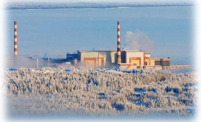
COLA Nuclear Plant
