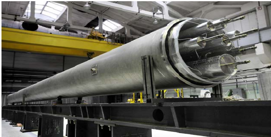
12-m section of the main helium pipeline for the XFEL (IHEP)
