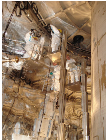
PMT installation inside Water Tank (May 2009)
