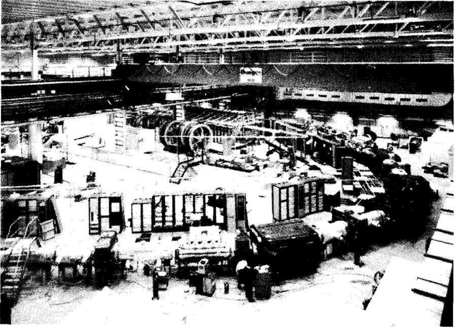
*Fig. 15.* View of the Antiproton Accumulator before it was covered by concrete slabs. The silvered material around the vacuum tanks is insulation, needed because everything may be heated to 300° to obtain ultra-high vacuum. The transmission lines crossing the ring and carrying the cooling signals may be seen.
