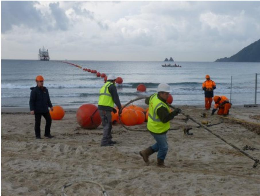
Main electro-optical cable deployed
