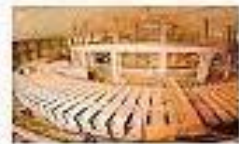
Synchrotron (shut down)
